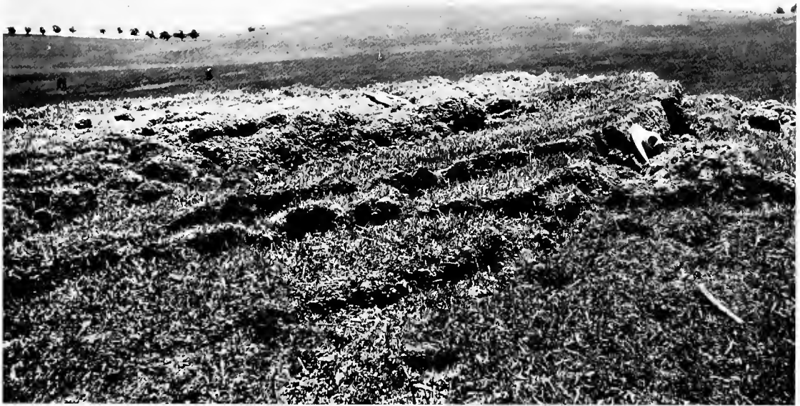
A. Concentric cracks in ground around an old alkaline spring, 1.5 miles north of Livermore. R. C.
